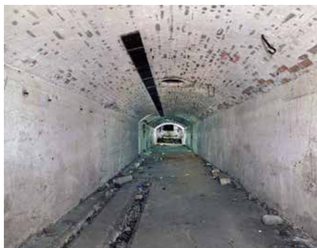
The bombproof shelter, the main entrance is to the right and the engine room is to the left. Photo Nick Catford
